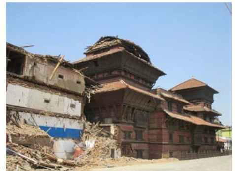
Damage of Kathmandu City (2 June 2015)
